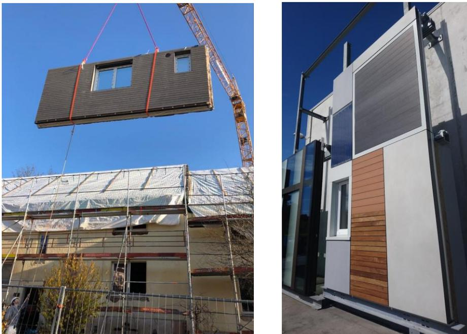
Abbildung 67 **Serielles Sanieren.** Links: Energiesprung [dena 2019]; Rechts: RenoZEB [Anonymus 2023b]
