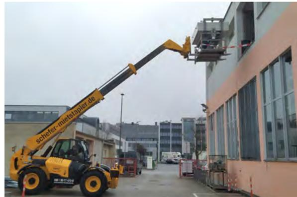
**The first dimensional stability furnace** is carefully lifted out of the building opening
